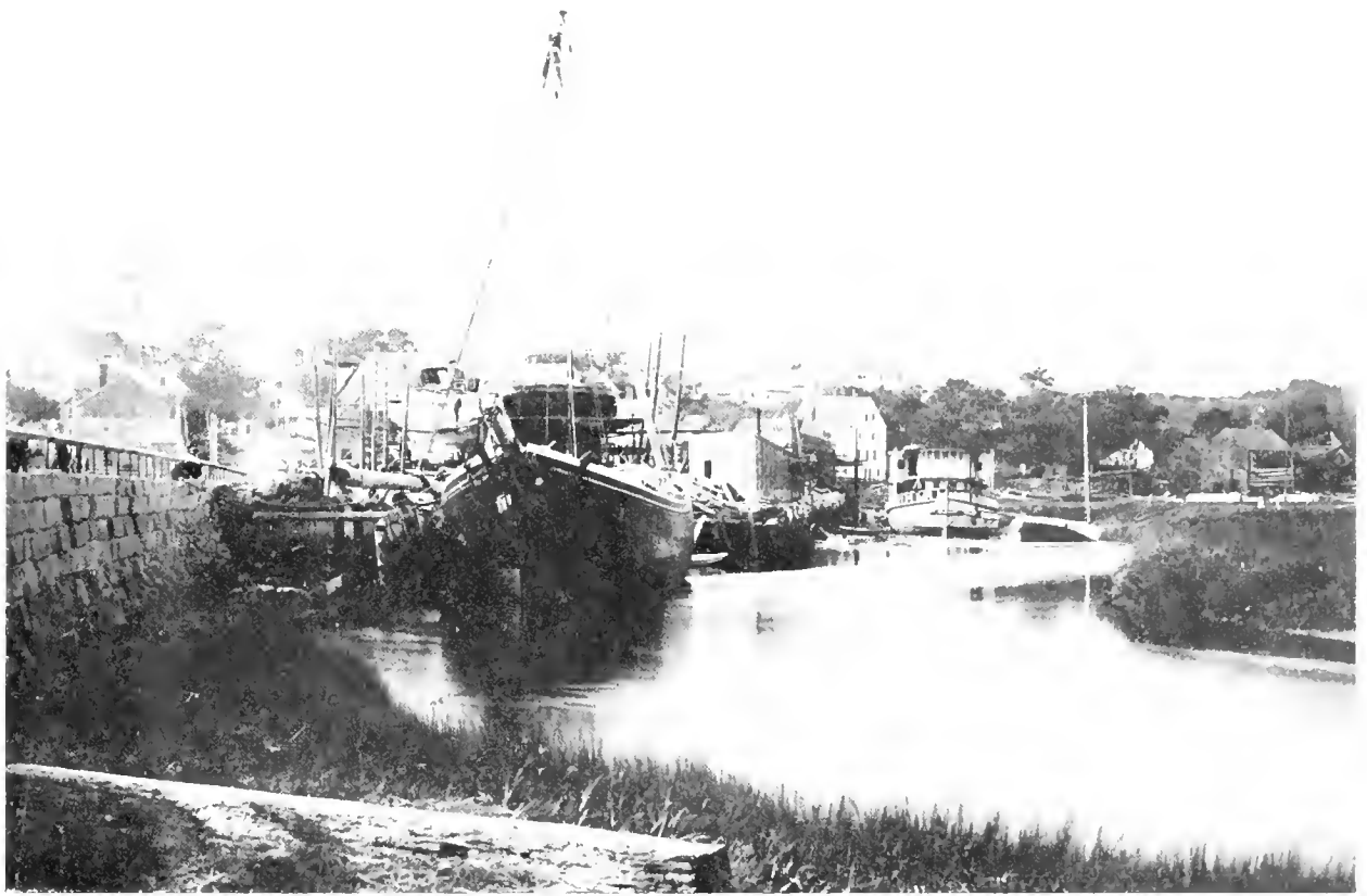
LARR AND JAMES SHIPYARD AT ESSEX, MASSACHUSETTS, ABOUT 1885, with one vessel in the water and another behind it on the ways. A new river steamer is in the background and other yards are beyond, with three ships on the ways. Center of village is to left, in background. Sheers and hoisting tackle are rigged to step the mainmast of the schooner in the foreground. The mast is alongside on the wharf. ( Smithsonian photo 44-9; h. )
